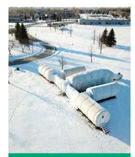
The Inflatable Lunar/Mars Analog Habitat (ILMAH) has five modules: the living quarters module, a botany/greenhouse module, geology module, exercise module, and an extravehicular activity (EVA) module. Docked to the ILMAH via a tunnel is the Pressurized Electric Rover (PER), which students used to conduct EVAs outside of the habitat.
