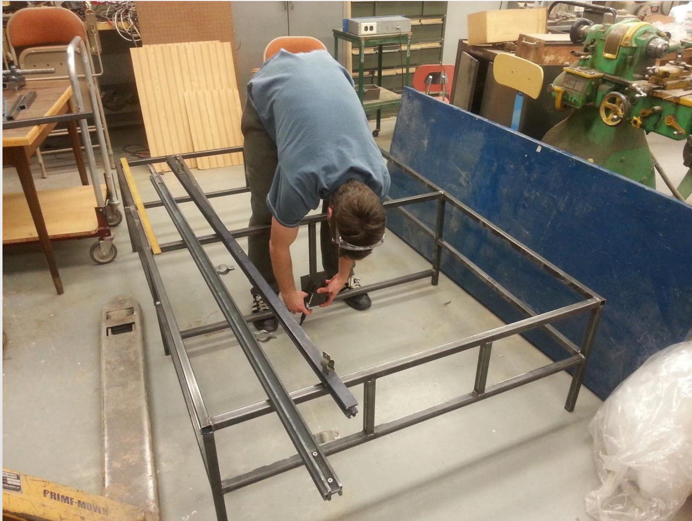
Placing the actuator mount.
