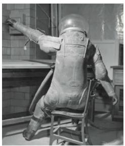
Figure-1 Goodyear Tire and Rubber Co. XH-3 prototype high altitude pressure suit (1943). Note: cable assisted shoulder joint.
